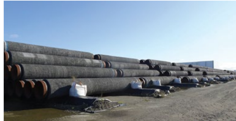
IMAGE: Pipes for the Nord Stream 2 (@Gerd Fahrenhorst)
